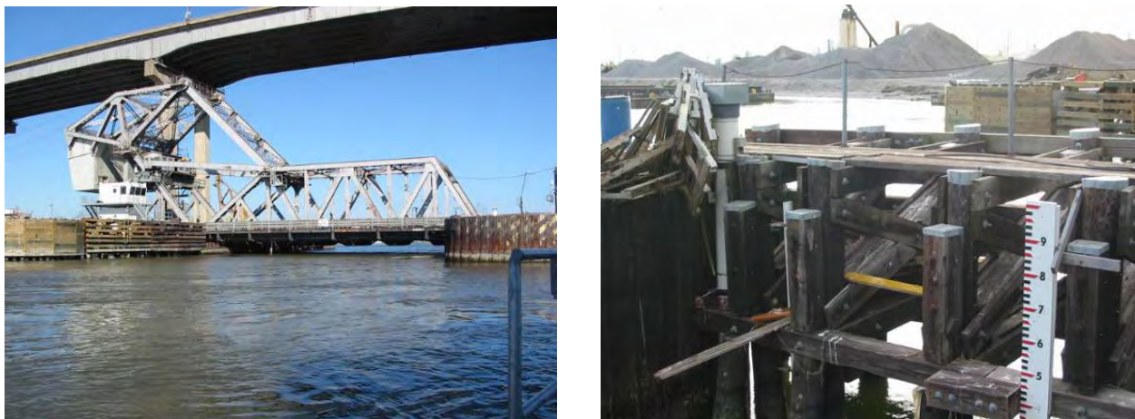
Figure 64. (Left) IHNC Almonaster Bridge—low chord elevation 3.51 ft NAVD88 (2004.65). (Right) Leveling to USGS recording gage and Orleans Levee District staff gage on I-10 bridge over IHNC
