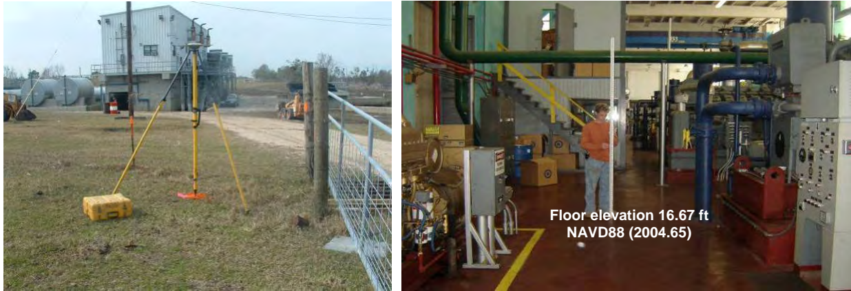
Figure 63. (Left) Static GPS survey to establish elevation on a benchmark outside a St. Bernard Parish pump station. (Right) Leveling first floor elevation inside Jefferson Parish Pump Station No. 3
